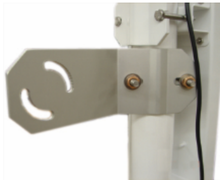
FIGURE 6-31. Antenna bracket mounted to pole
