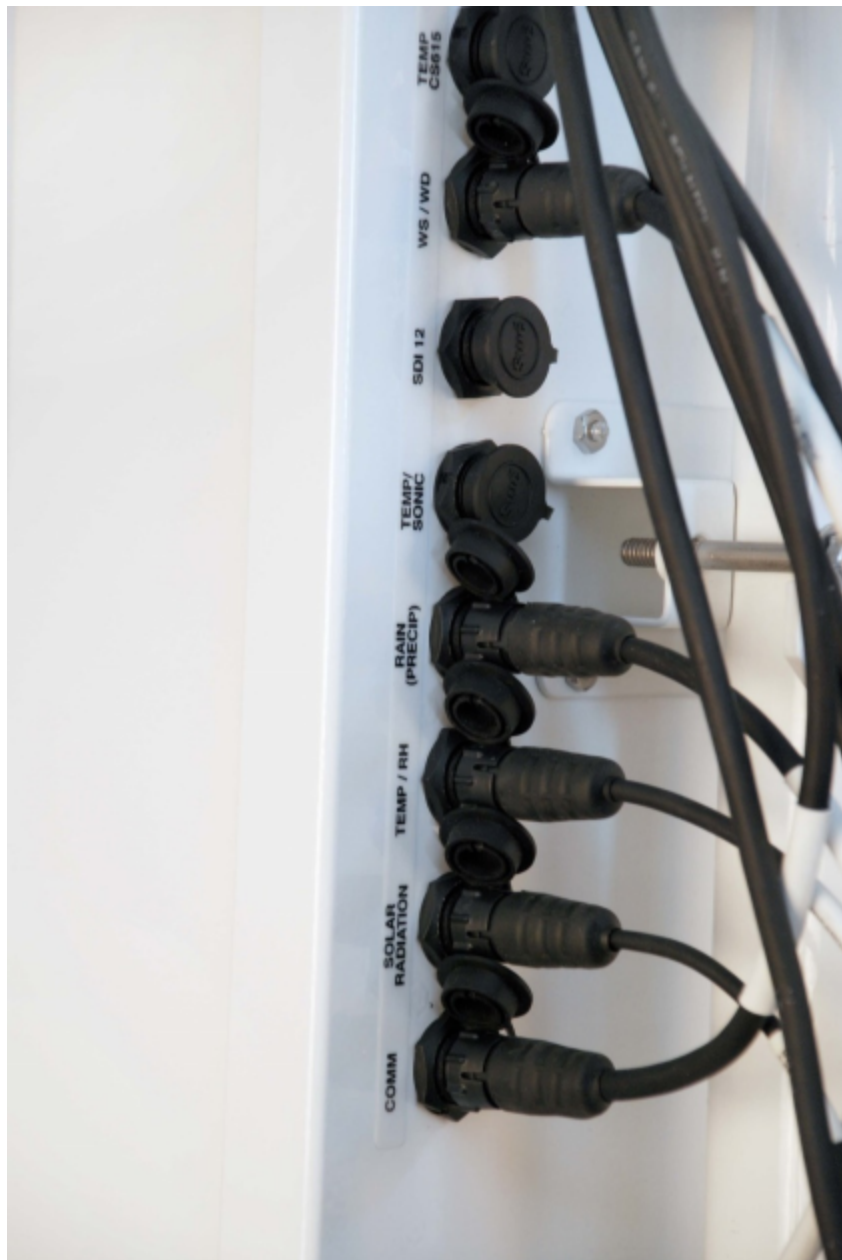
FIGURE 6-21. Connecting sensor cabling to enclosure
