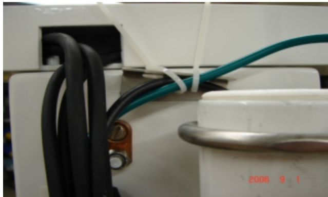
FIGURE 6-28. Loosely wire tie antenna cable
