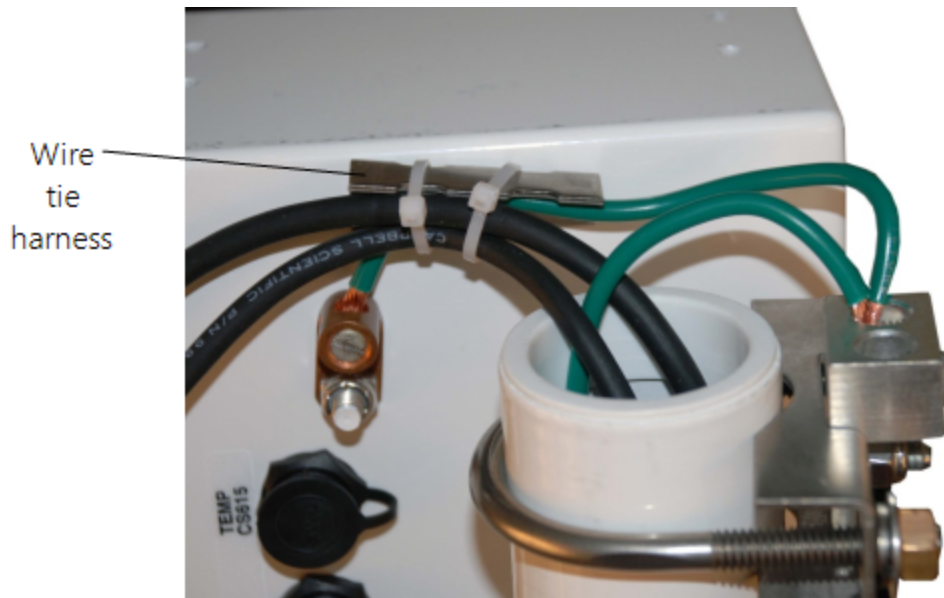
FIGURE 6-46. Cabling strapped to wire tie harness
